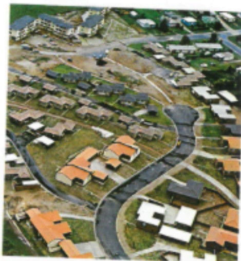
1970 — New housing subdivision
