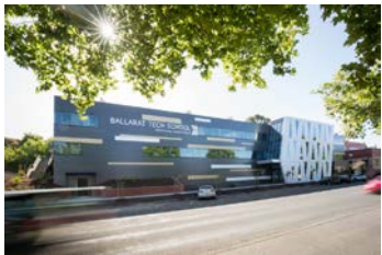
Ballarat Tech School Building K, Albert St
