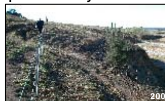
Looking downstream - Installation (Photo C. Massey)
