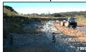
Looking downstream - Installation (Photo C. Massey)
