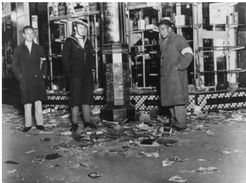
Pickets and broken windows Queen St April 14 th 1932
